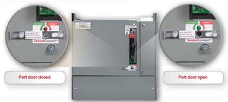
**Actuator Position Indicator and Tool Insertion Point**
